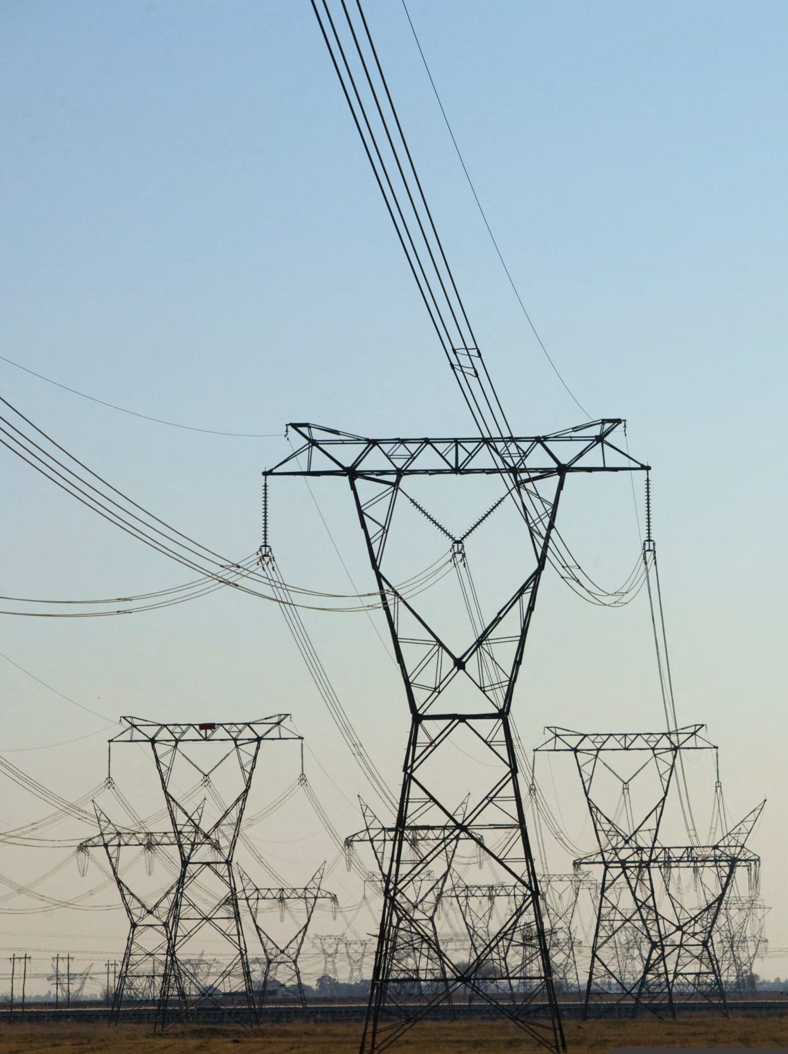
The Lethaba Power Station outside Sasolburg in the Free State.
